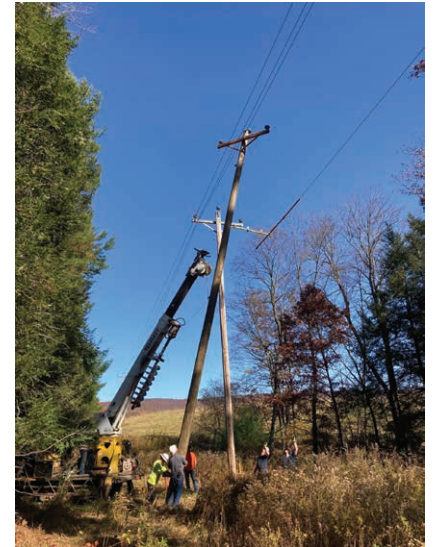
POLE REPLACEMENT: New Enterprise REC lineworkers use a track-mounted digger while replacing a pole in a remote area of Sherman's Valley.
