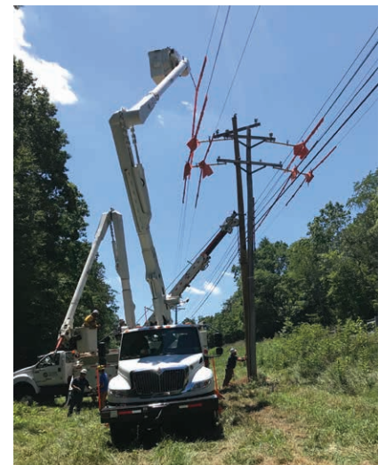
POWER BEHIND THE POWER: New Enterprise REC lineworkers replace a pole carrying two separate circuits along Waterfall Road in Three Springs.
