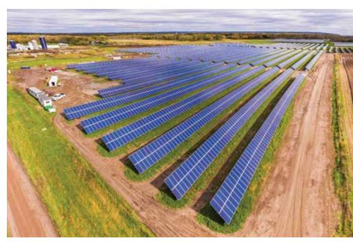
CPV Maple Hill is a 100-MW solar farm in Portage Township, also in Cambria County. According to a press release on the CPV website, the facility occupies more than 700 acres with the ability to power 18,000 homes. The power-density number for this project is 0.14 MW per acre.
